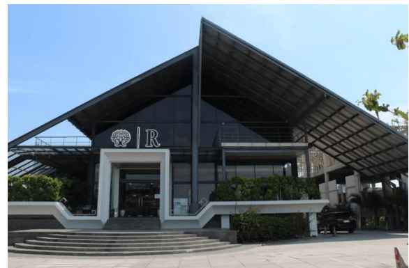
Figure 6. Facade of El's Coffee Roastery Building
