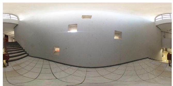
Figure 6. Panoramic Picture in Stairs Area.
